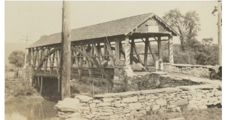
CATOCTIN CREEK BRIDGE
